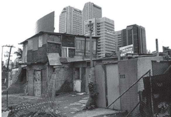
FIGURE 4 – The reutilization of the discarded material in the construction of slum sheds. São Paulo. Source: Geoff de Verteuil, 2003
